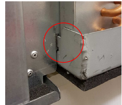
Fig 8.2b: Drain Tray Rear Support Lugs
