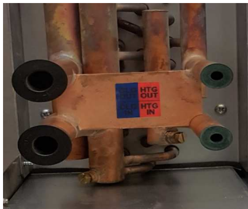
Figure: 5.4a Identification of heat exchanger coil connections
